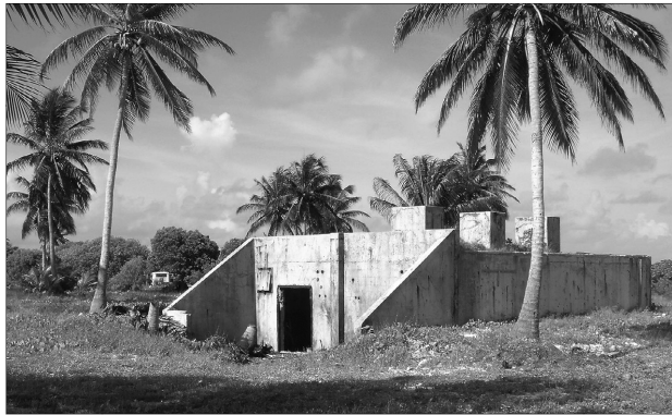
Figure 7: Reinforced concrete blockhouses, such as this former electrical generator building on Eneu Island at Bikini Atoll, often took numerous forms. The two wing walls extending from the building's front face allowed for sand to be mounded up against and on top of the structure for increased protection from explosive damage and radiation.
